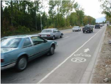
The ideal (and statistically safest) on street bicycle route is the designated bike lane however shared lanes can be designated where space for a dedicated lane is not available.
