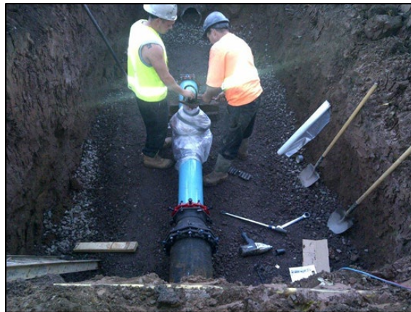
Figure 5: Water Main Valve Installation
