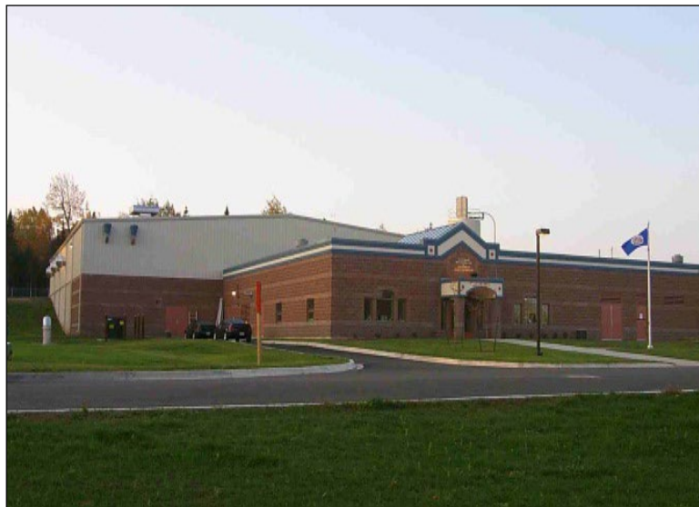
Figure 3: Moncton Water Treatment Plant
